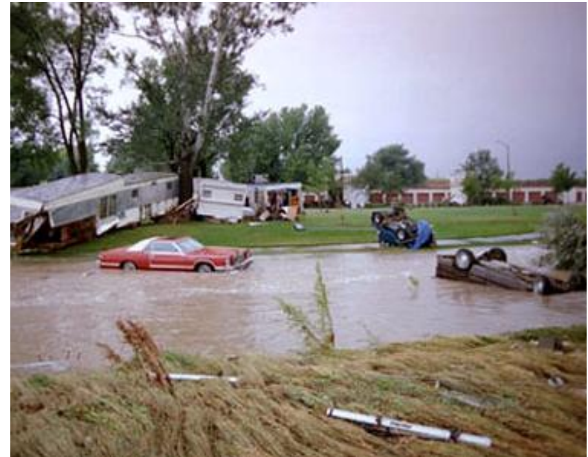
Damage along Spring Creek after a flash flood in Fort Collins, Colorado (July 1997)
